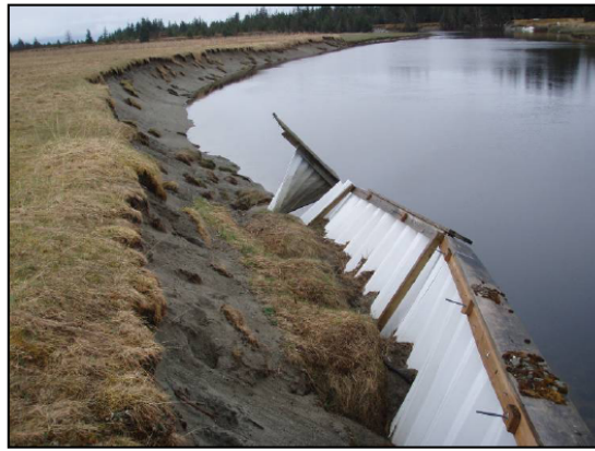
Figure 4: Downstream end failure of sheet pile
