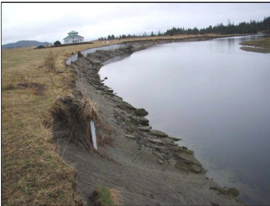
Figure 3: Upstream end scour of sheet pile
